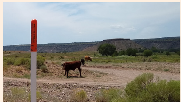
Middle Rio Grande Pueblo fiber marker near San Felipe Pueblo connecting to Santo Domingo Pueblo follow pre-disturbed back roads to minimize the environmental impact of the fiber route.
