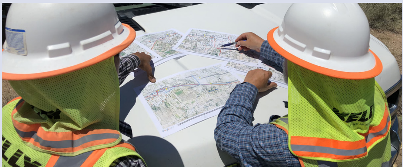
Kelly Cable of NM crew reviews route maps to complete the final 12-mile stretch along NM State Highway 550.
